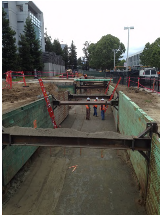
A Sliding Shoring System without Rail Posts
