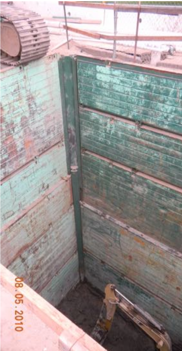
Telescopic Slide Rail Shoring: 35' Deep.
