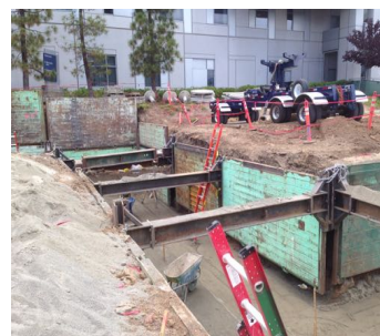
Hydraulic Trench Shield: very high clearance, 'MAXSHORES'.
