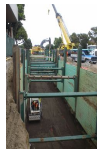
Hydraulic Trench Shield: very high clearance, 'MAXSHORES'.
