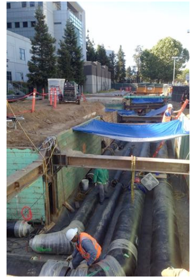
Project: Sliding Strut Shoring System. NO RAIL POSTS
