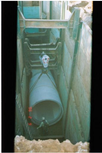
Slide Rail Unique Panel : Trench 75'x11' @ 32' deep in cobblestones.
