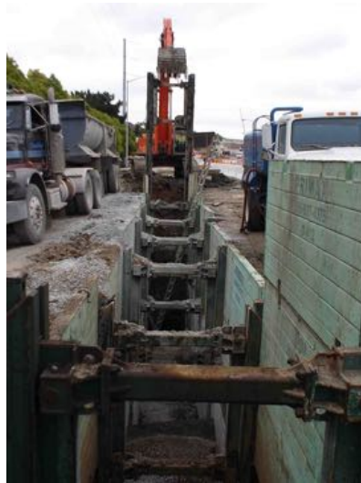
Slide Rail: Trench 65'x4' @20' deep in Bay Mud.
