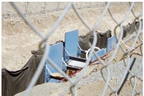
Hydraulic Trench Shield: very high clearance, 'MAXSHORES'.
