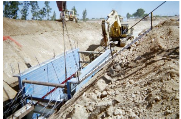
Trench Shields: two stacked 36' long x 13 ft wide x 10" wall
